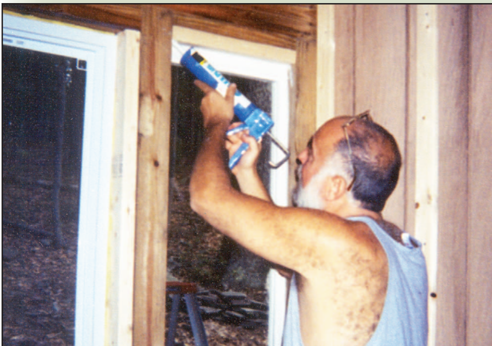
Installing and caulking an odd-sized piece of glass created a window.
