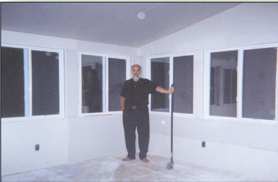
The room is ready for spackling.
