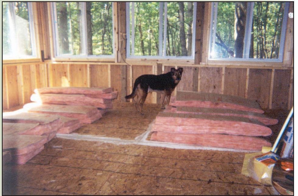
The late, great Zeus inspected the framing and insulation.
